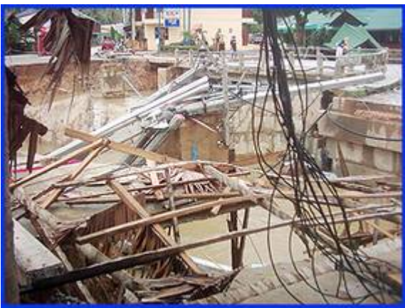
This used to be a bridge.
